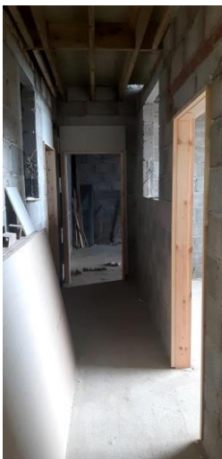
The image shows the door frames which were fitted in all of the Madrasah classrooms.
