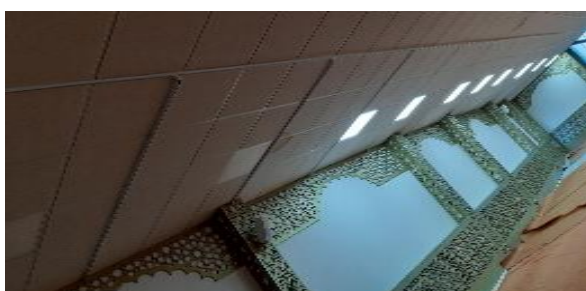
The image shows the Itekaf cubicle curtain tracks which were installed in the main prayer hall of the Mosque.
