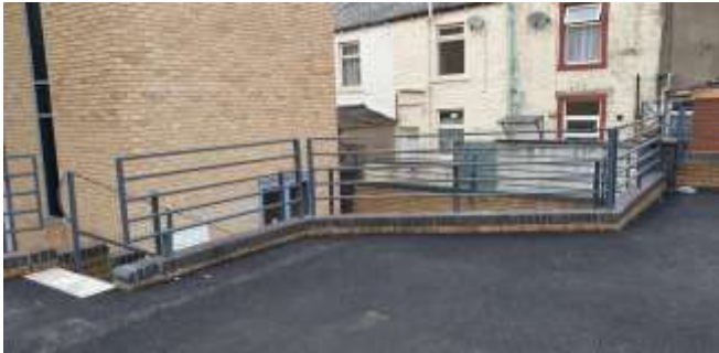
The image above shows the safety railing installed on the retaining wall.
