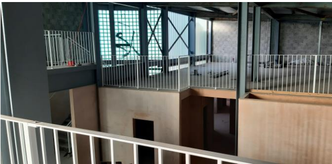
The image shows the painted steel pillars on the first floor.
