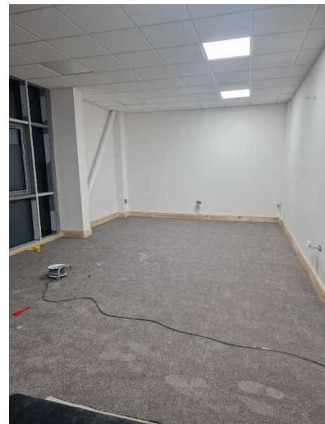
The image above shows the first floor conference rooms suspended ceiling fitted.
