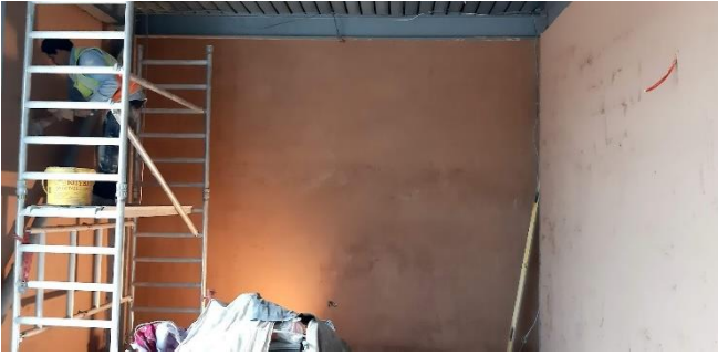
The image above shows the plastering of the first floor classrooms.
