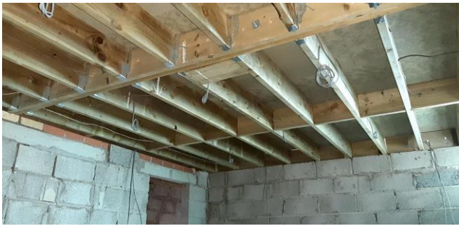
The image above shows the ceiling which was constructed for the Madrasah classrooms.
