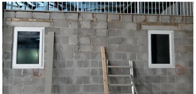
This image shows two of the double glazed windows which were fitted in the Madrasah classrooms.
