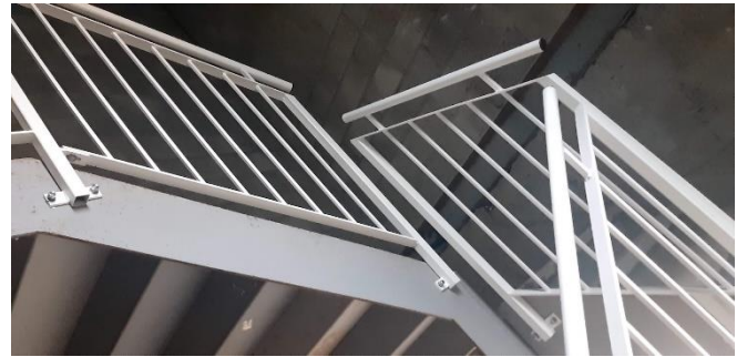
This image shows installation of First floor rear stair railing.
