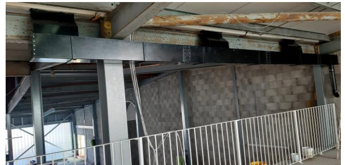
The image shows the newly fitted Gutter on the first floor.
