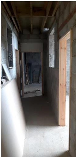
The image shows the door frames which were fitted in all of the Madrasah classrooms.
