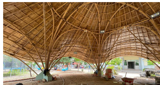
Internal view of bamboo roof canopy structure
