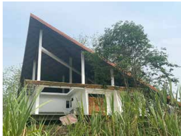
Overhanging roof to give shade and protection
