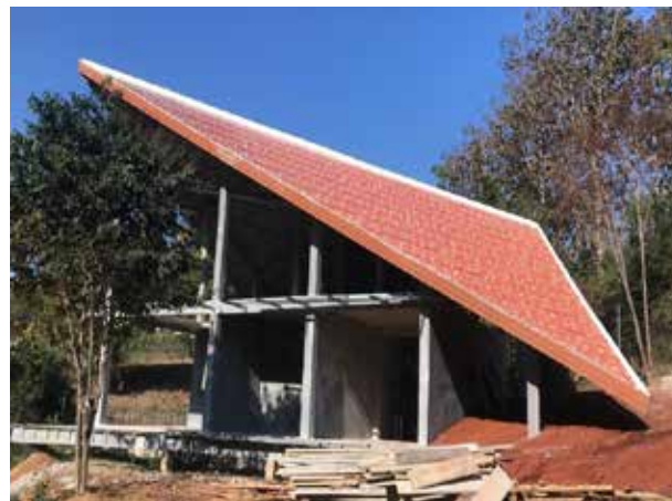
Overhanging roof to give shade and protection
