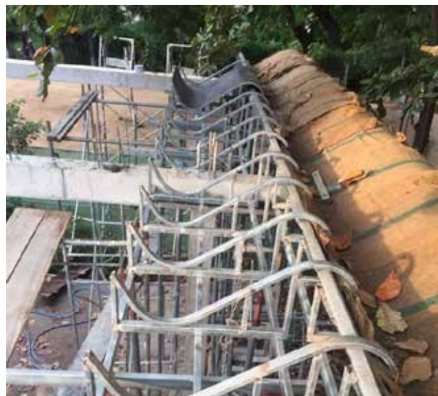
S curve elements to create roof
