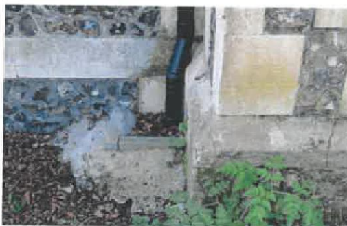
13. Gully to north aisle filled with leaves.
