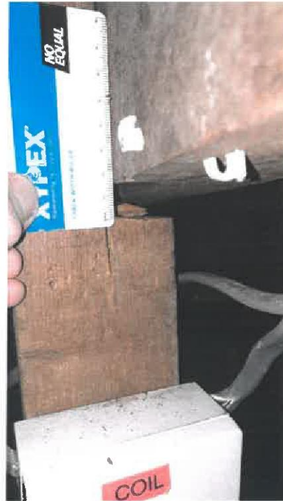
Photograph 3: 15mm vertical settlement between timber post on internal sleeper wall and floor joist.
