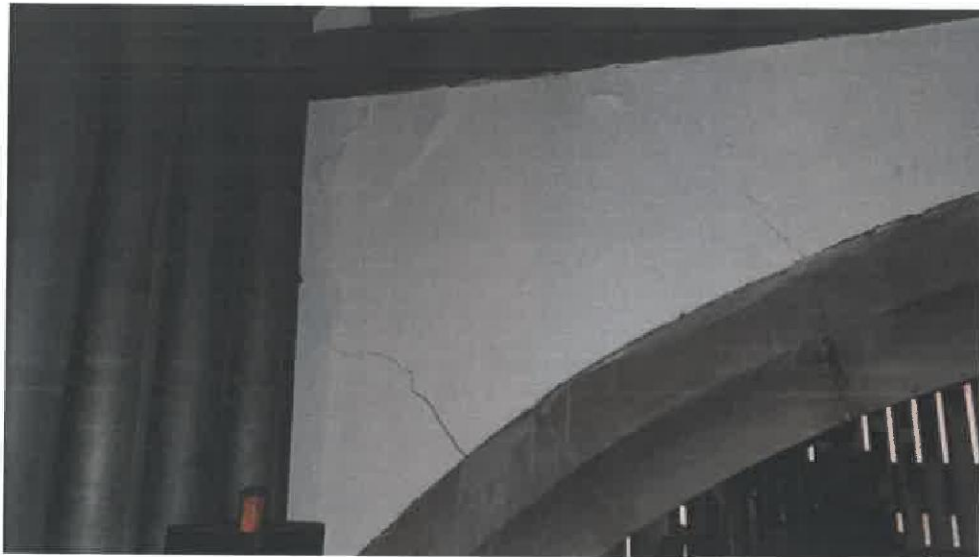
Photograph 7: Cracks from within organ loft of arch into the chancel area.
