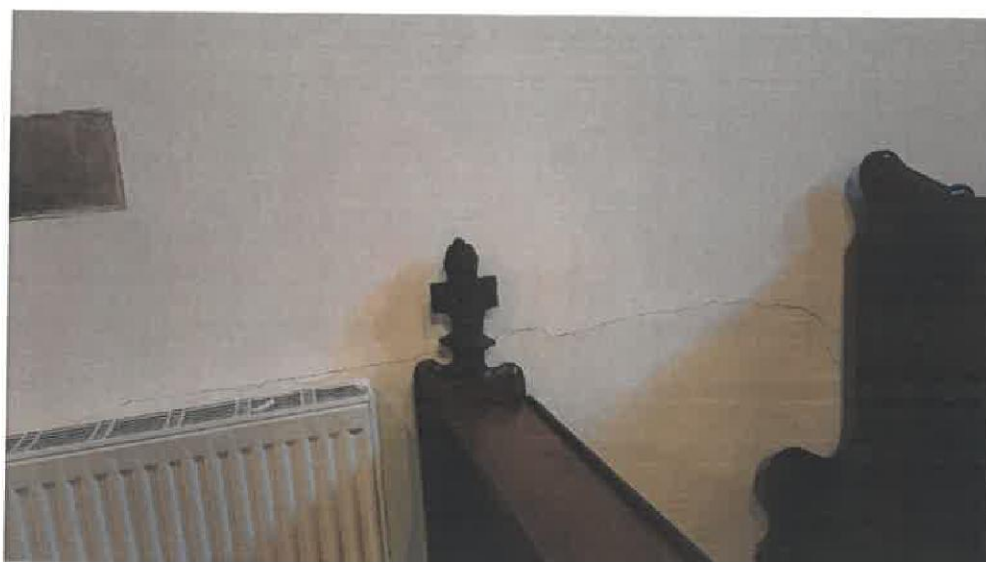
Photograph 8: Horizontal cracking to north aisle external wall
