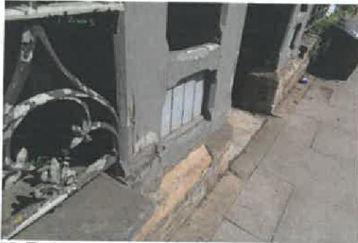
25. Timber decay to the exterior of the lych gate.
