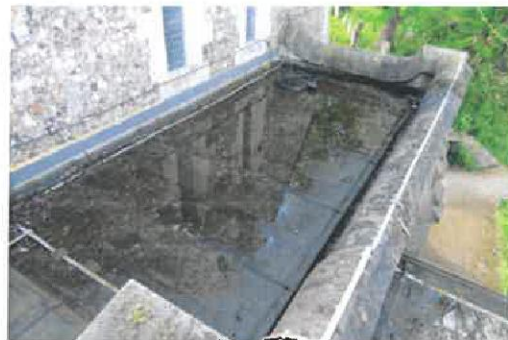
6. Ponding to small flat roofs.
