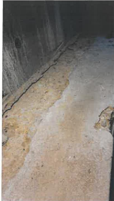
Photograph 1: Cracking between the RC ground beam and ground bearing concrete upstand indicating differential settlement.
