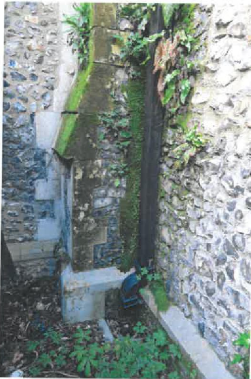
11. Saturated masonry of the buttress at the east end of the south aisle.
