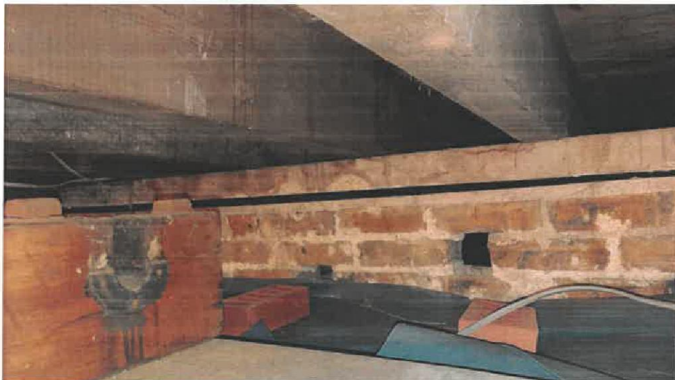
Photograph 2: Sleeper wall has settled allowing a gap to form under the timber wall plate
