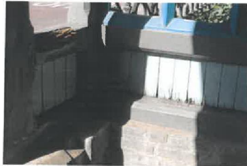
26. Timber decay to the interior of the lych gate.
