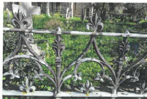
22. Peeling paint to front boundary.
