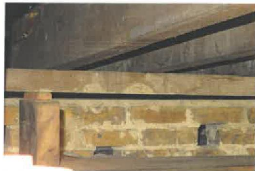
4. Gap appearing above the brick sleeper wall which no longer supports the joists above.
