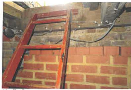
16. Trailing cables beside ladder to chamber below organ.
