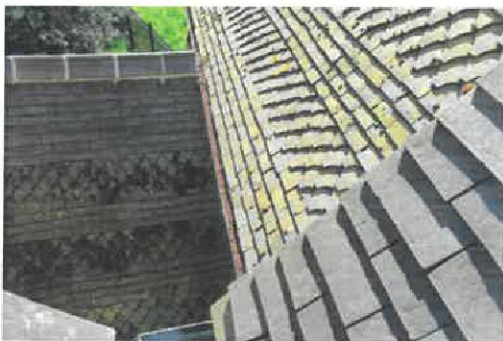
7. Blocked gutter to north side of chancel
