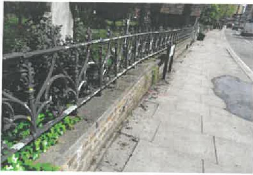
23. Movement in the front boundary railings.
