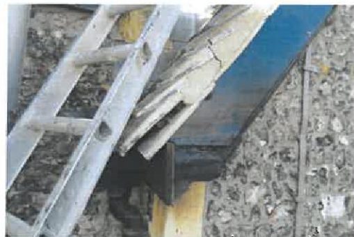
8. Access ladder damages the NW corner of the nave roof.
