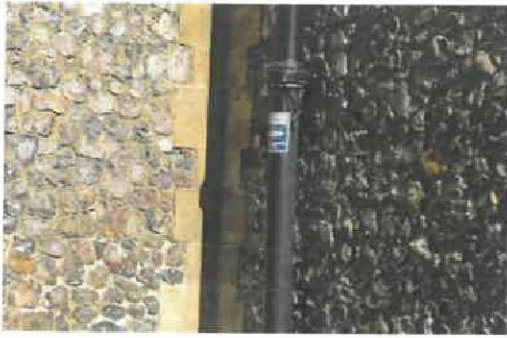
15. Cracked downpipe to south side of organ chamber.
