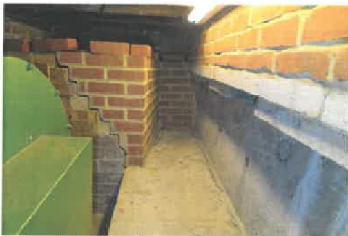
3. Chamber below the organ. Blower on the left. Settlement of ground supported structures.
