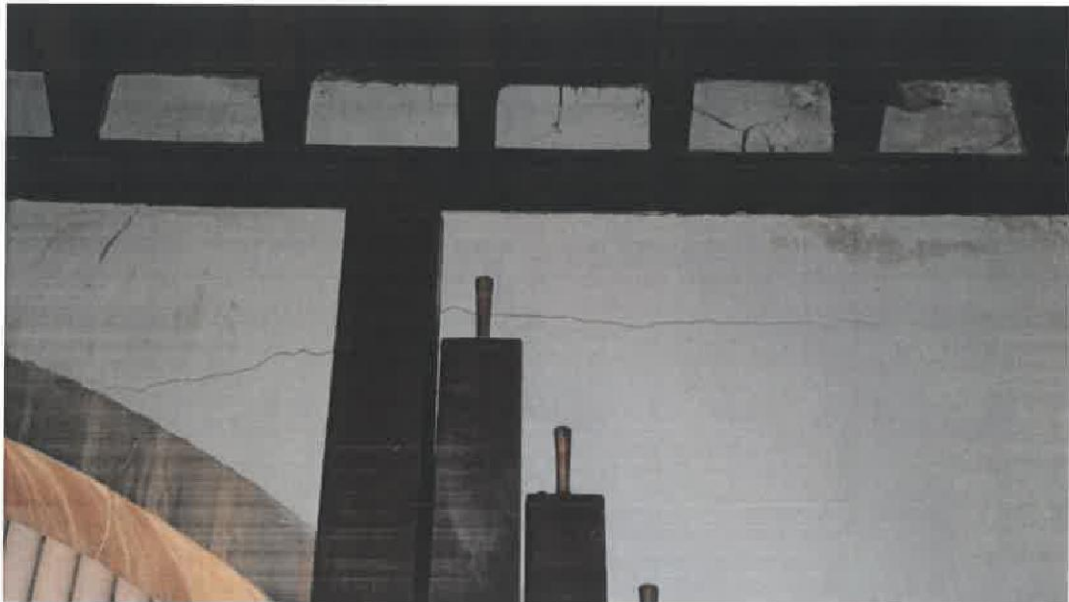
Photograph 6: cracking to south aisle wall from within organ loft.
