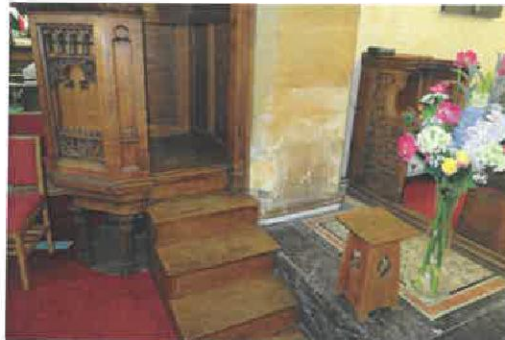
18. Evidence of saturated masonry behind the pulpit.
