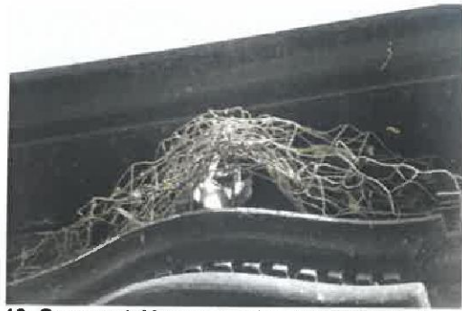
10. Ornamental hopper on the south side of the south aisle provides a nesting box for pigeons.
