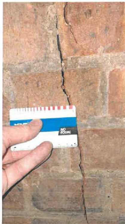
Photograph 4: vertical cracking to the internal sleeper walls to the undercroft.
