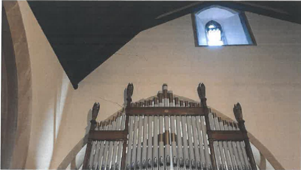
Photograph 5: Cracking above the arch between the south aisle and organ loft.
