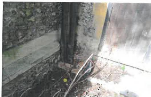
14. Gully to vestry filled with leaves.
