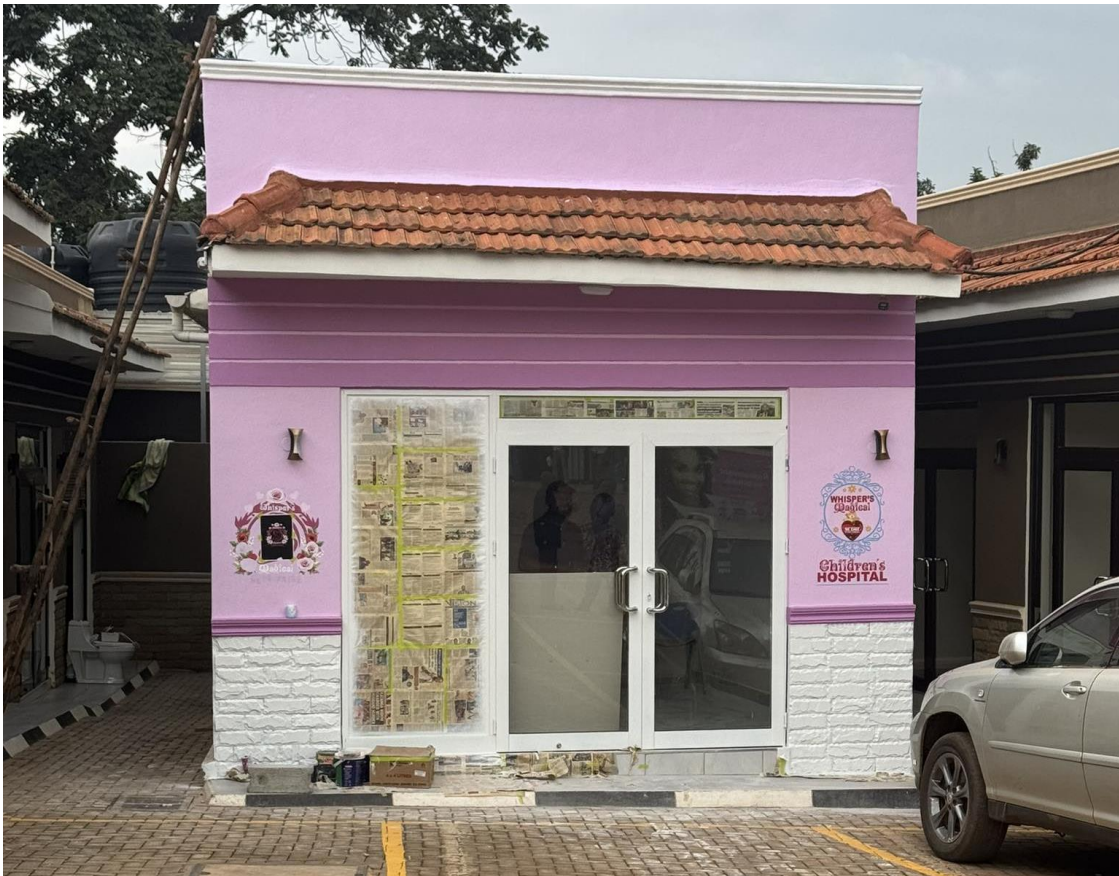
Whisper's new Kampala branch being fitted out
