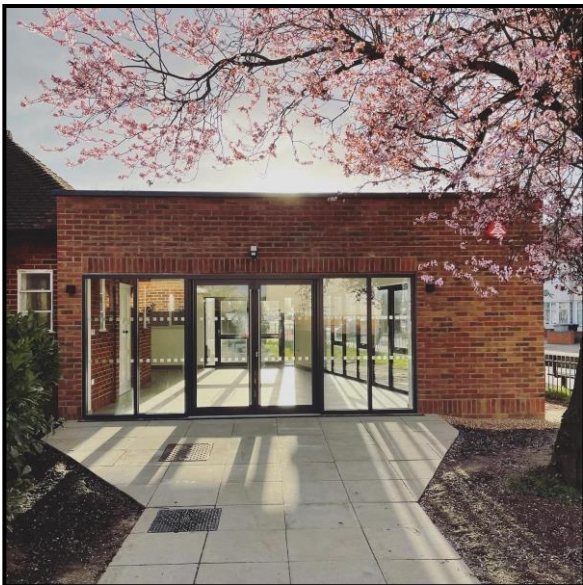
Roe Green Hall, Kingsbury extension
