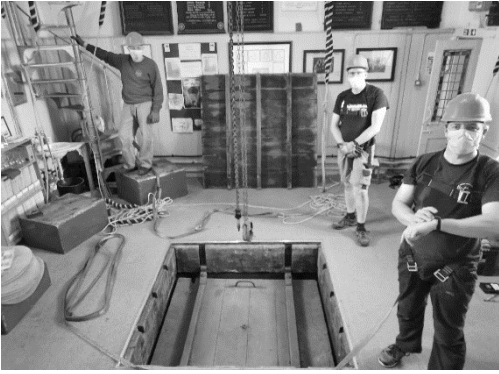
Lifting the trapdoors to bring the new wheel up the tower
