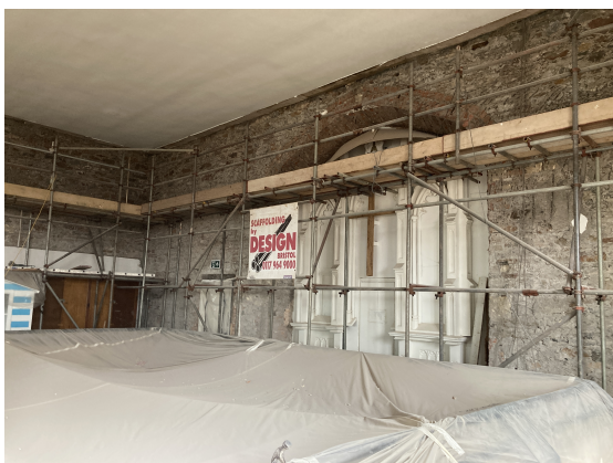
Example of the damage to the internal plaster
