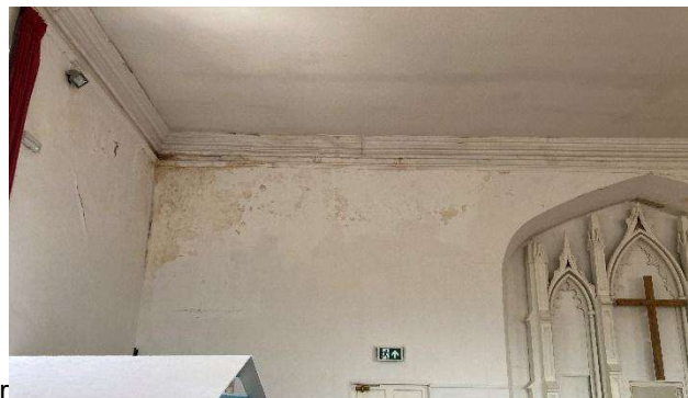
Example of the damage to the internal plaster
