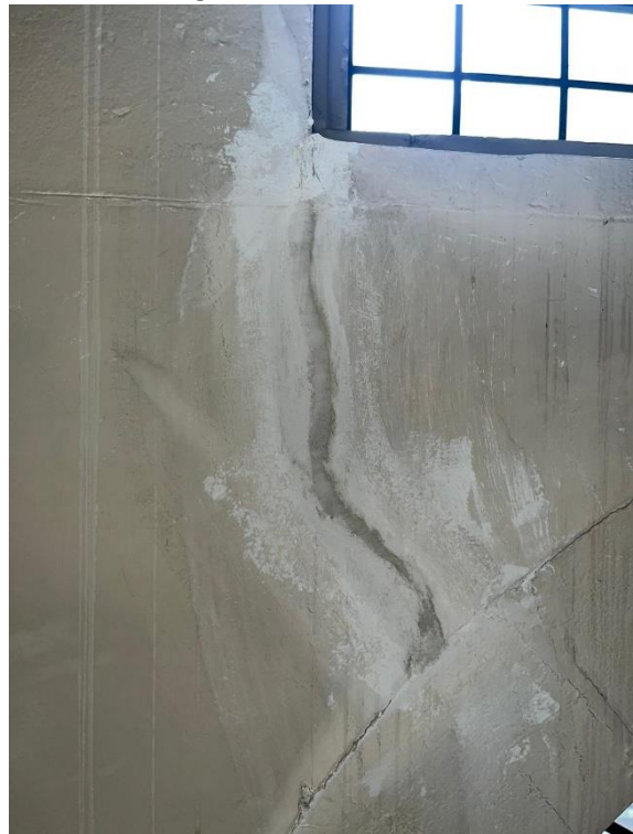
Repair of cracks
