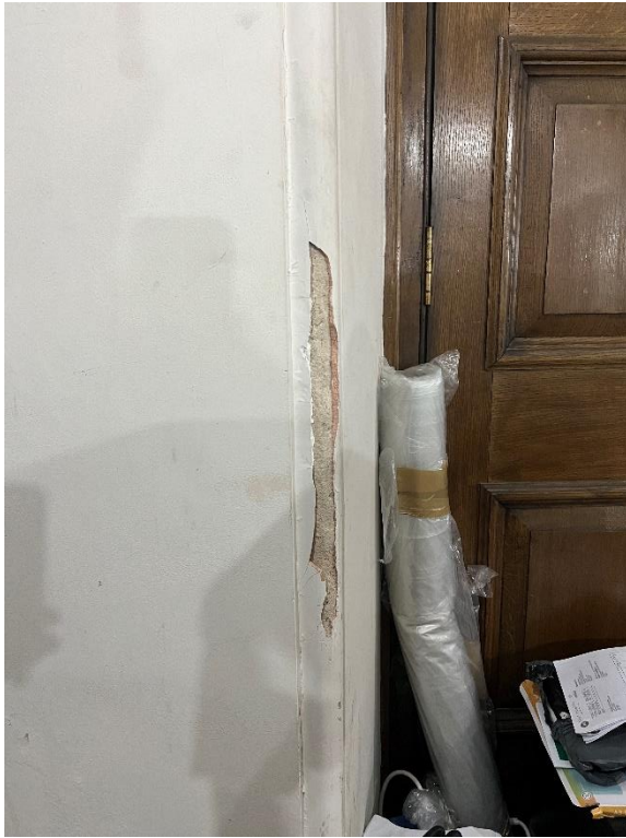
Repair damaged plasterwork
