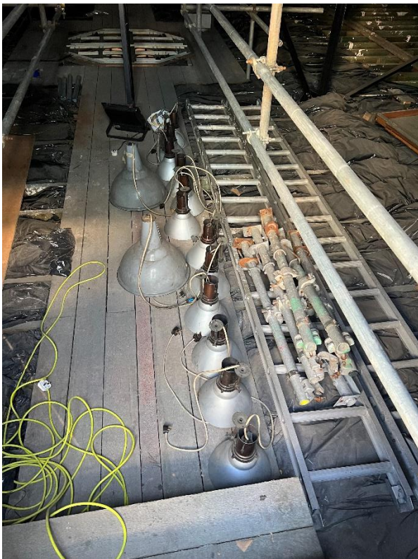
Removal of old lighting from roof space
