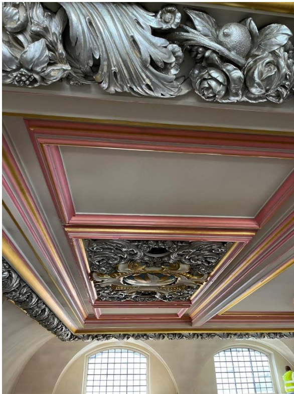
Cleaning the ornate ceiling mouldings
