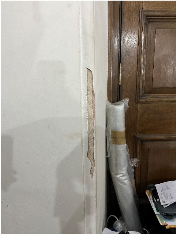
Repair damaged plasterwork
