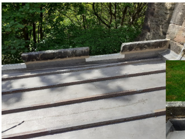
Picture 2 & 3 – additional weather detail between castellations
