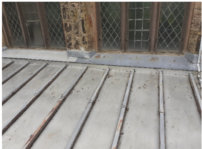
Picture 1 – weather shielding fitted to prevent driving rain being blown up and under roof sheet
