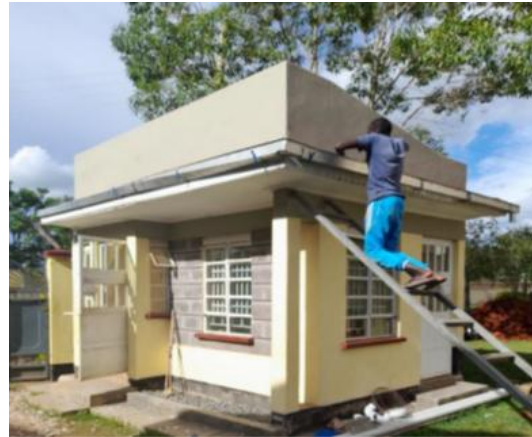
Completed Agro- business facility
