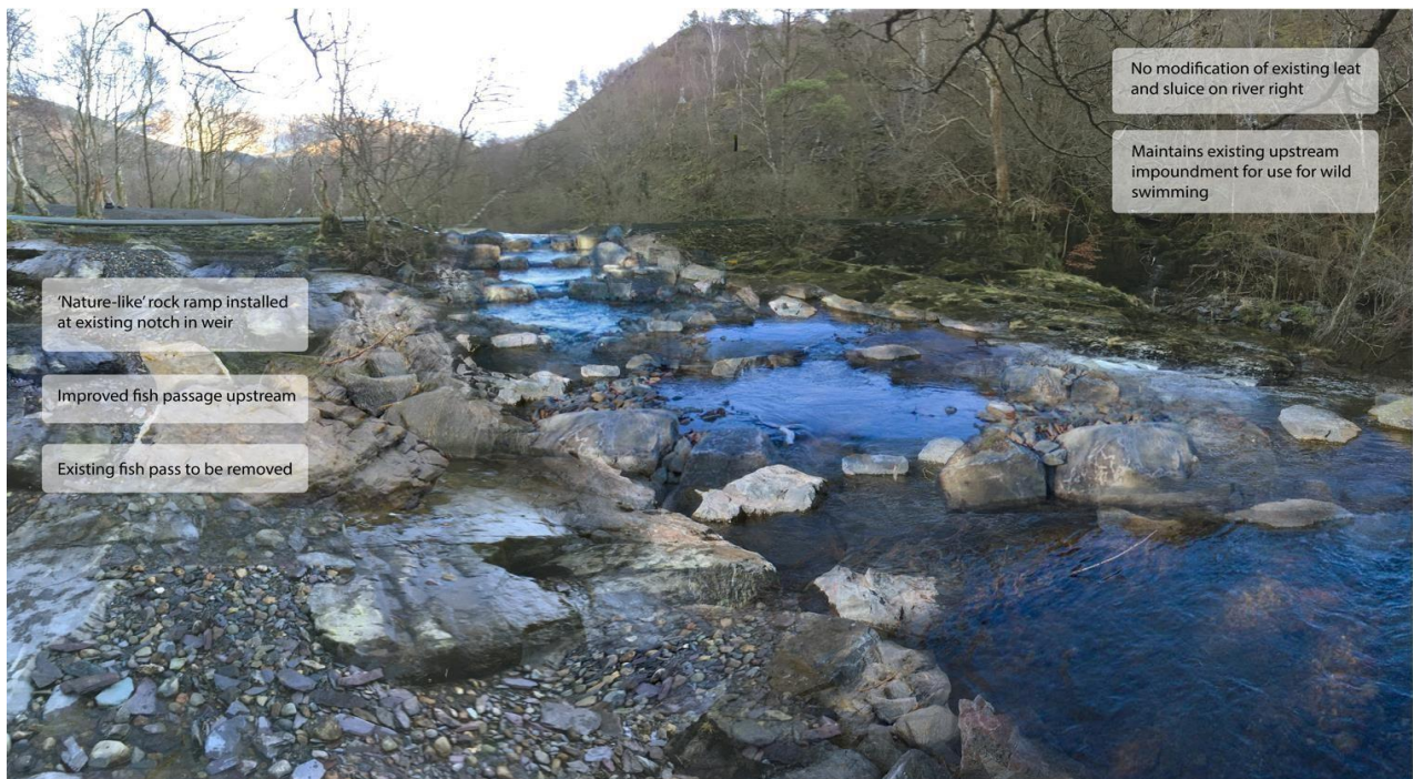
Current Weir showing fishpass not working
