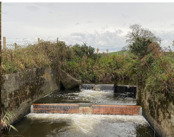
Weir with notch and removable timber pre-barrage
