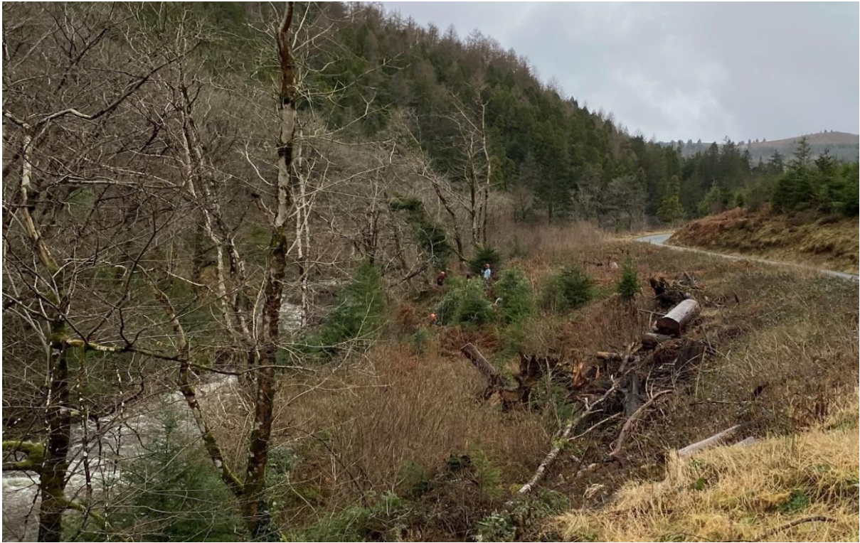
Contractors removing the trees within the project area
