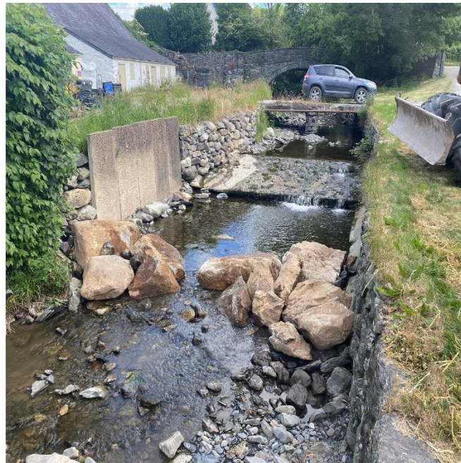
Pre – barrage Construction
