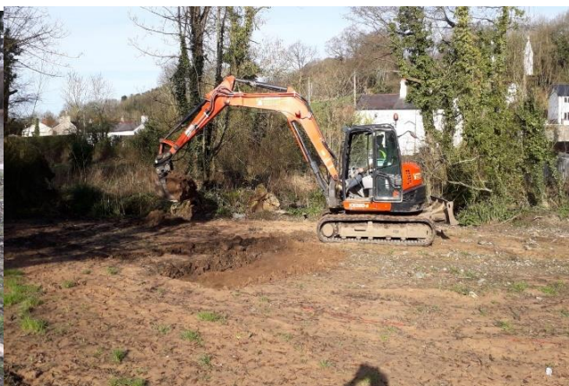
During landscaping works
