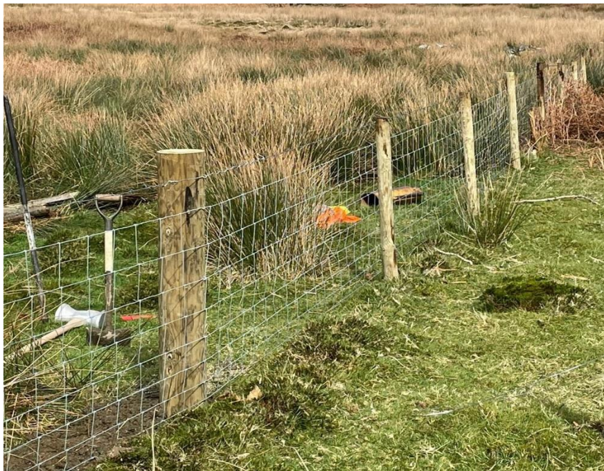
Repairs to the upper moorland fence line.
