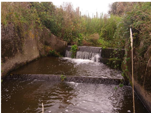
Weir Before work
