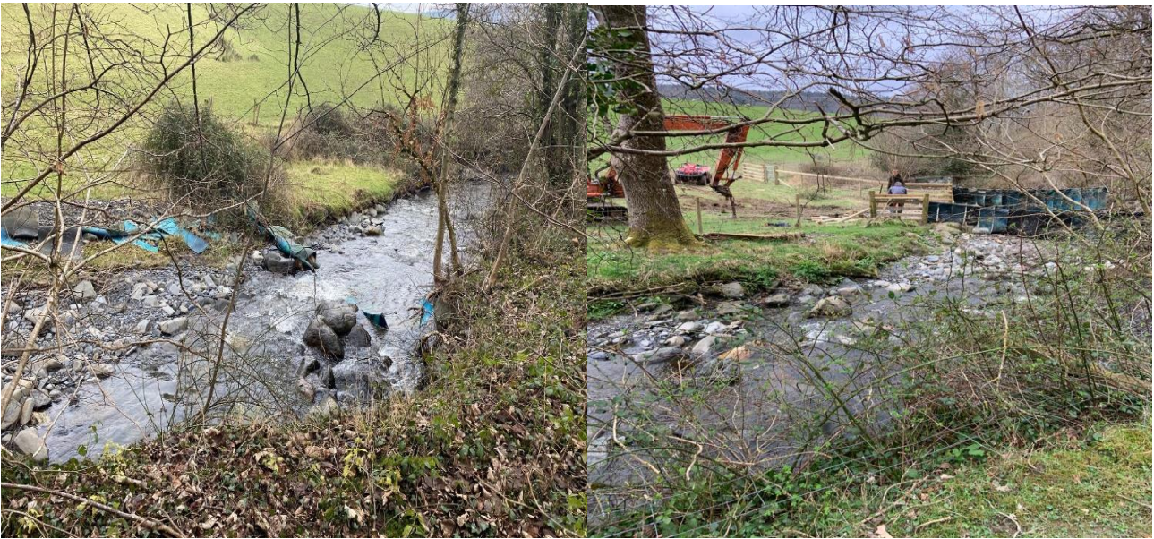
Old drinking bay destroyed by flooding
