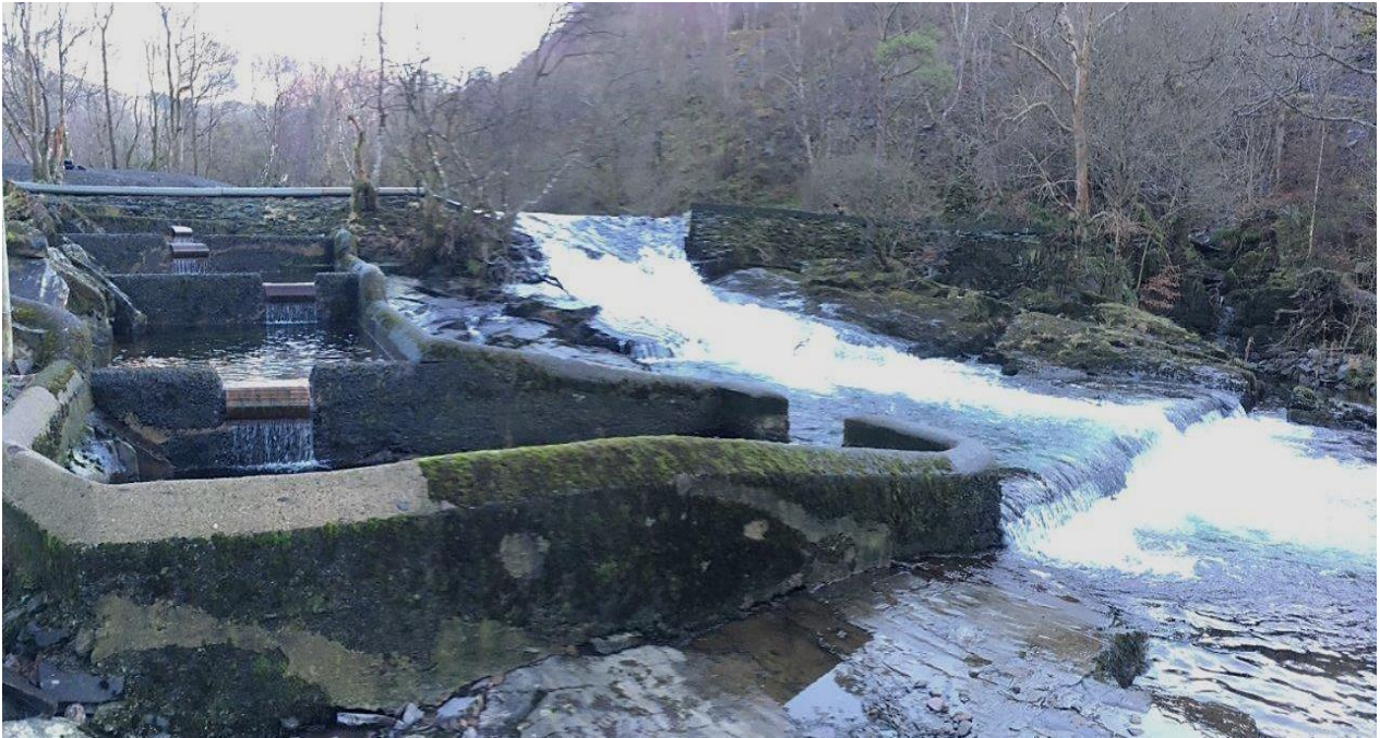
Current Weir showing fishpass not working
