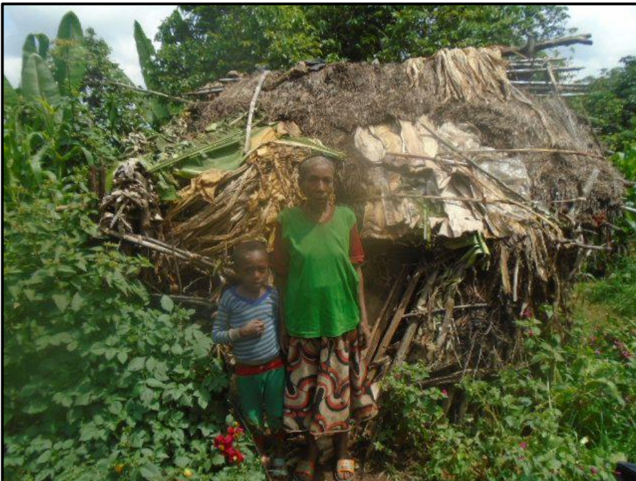
Unsuitable and unsafe dwelling 2022
