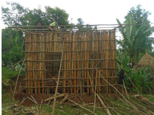
A house under construction.
