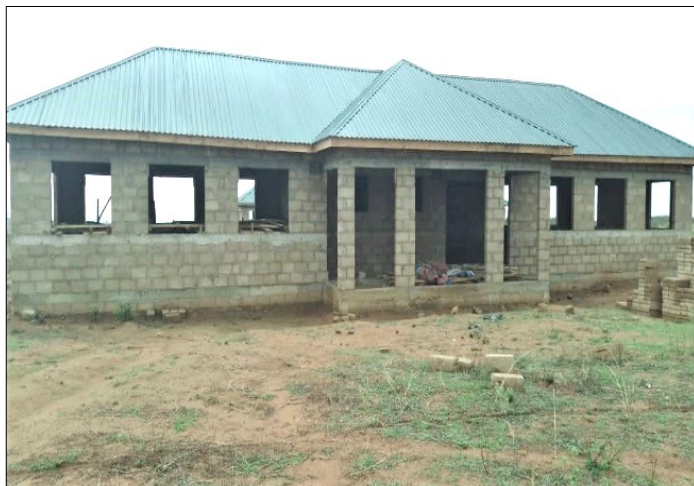
The roofed laboratories in December 2021. Since then, the walls have been plastered and doors and windows have
