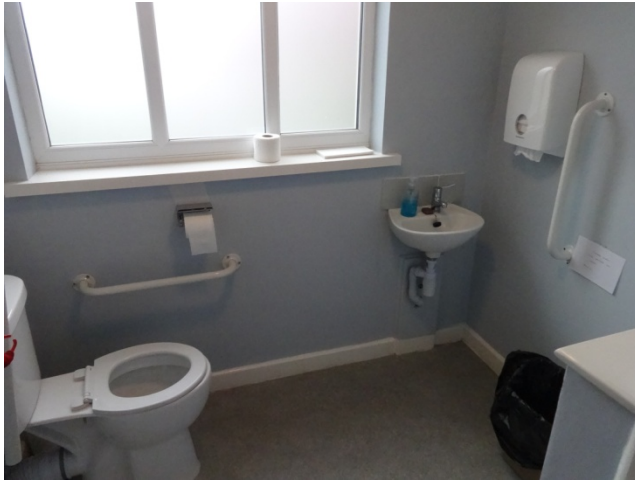
Storeroom converted to Disabled Toilet
