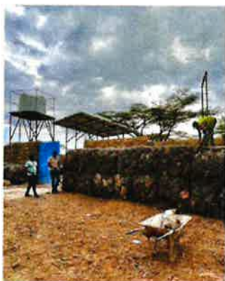
Reinforcing the new wall in Daaba after elephants repeatedly broke through the structure. © Jane Wynyard
