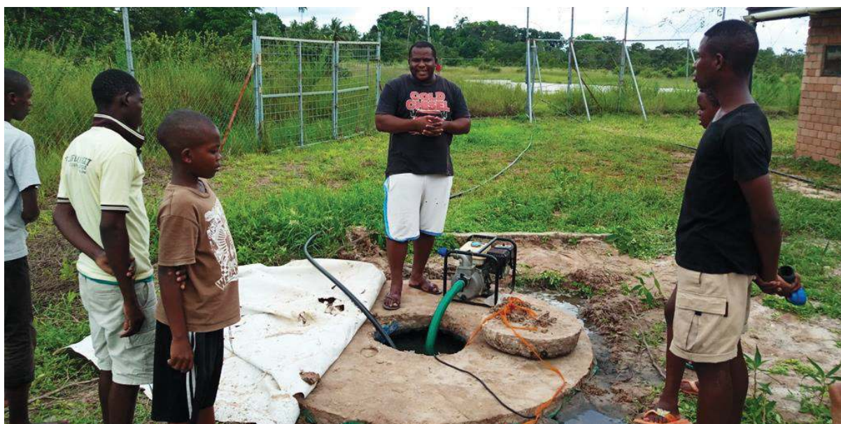
Fixing the water pump
