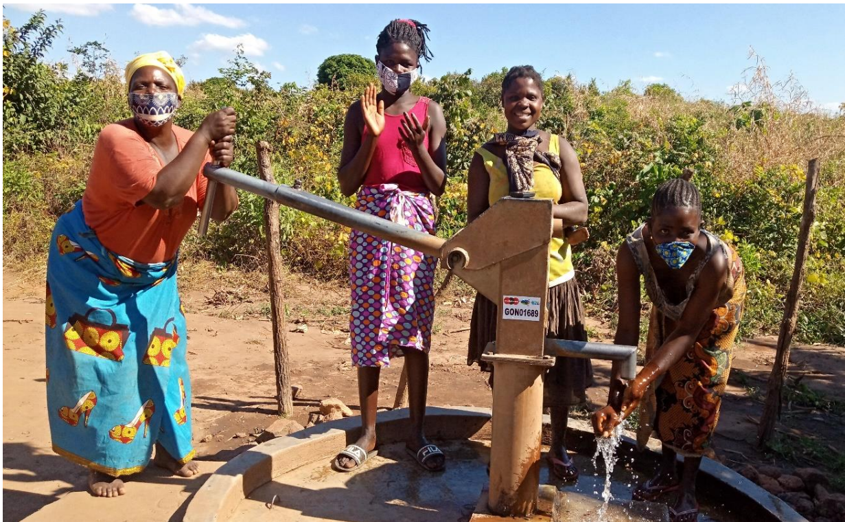
The newly repaired waterpoint in Nhaurunharu, Manica Province, Mozambique
