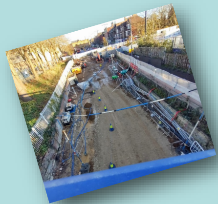
Botley Road bridge works
