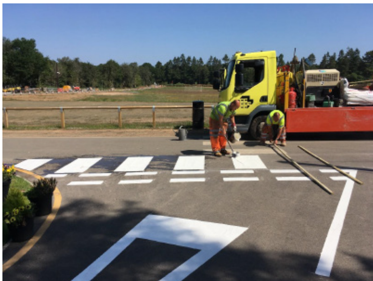
Line marking in progress
