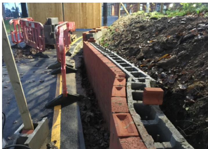
RC/Masonry retaining wall in progress
