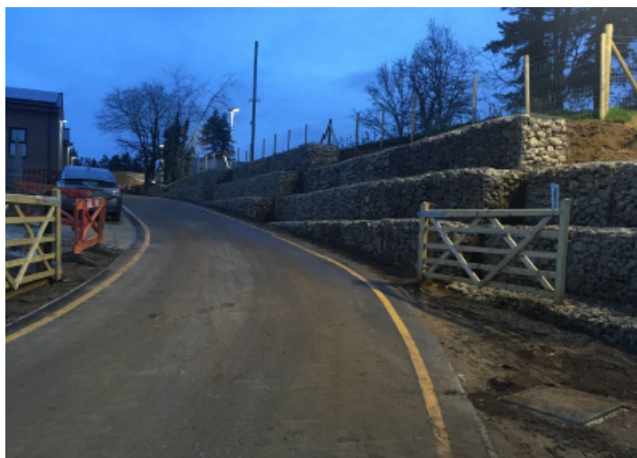
Retaining wall built using Gabion baskets
