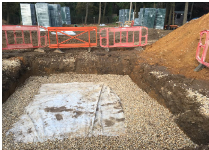
Soakaways construction for the road drainage system
