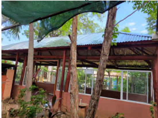
3 Refurbishment in progress using zinc sheeting
