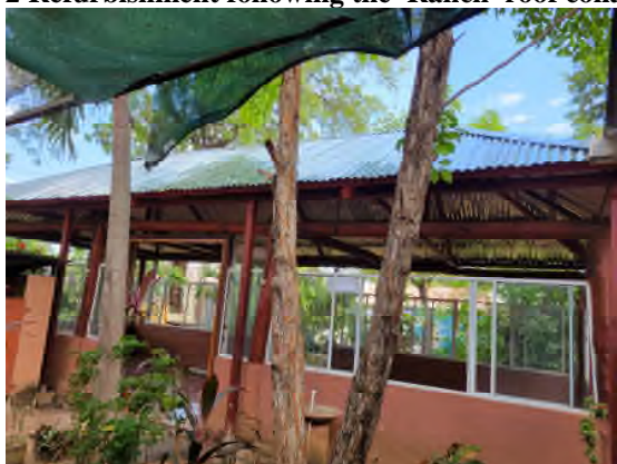
3 Refurbishment in progress using zinc sheeting
