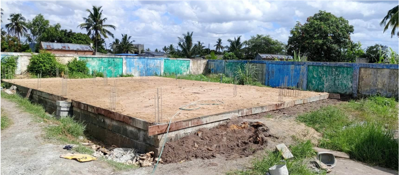
Completed foundations and base slab – November 2023
