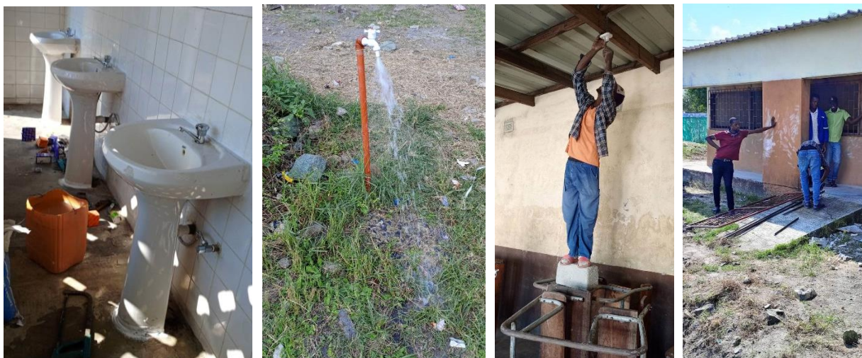
Plumbing repairs, electrical wiring, welding for security grills & pump housing
