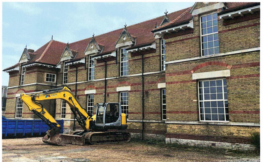
Building works at Victoria Barracks
