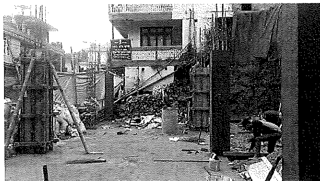
New RIBS School Facility in progress
