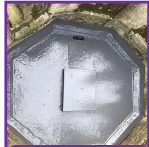
Two Tower Repair £12,374
