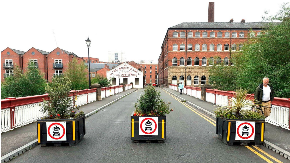
Ball Street Bridge, temporary closure soon to be made permanent and a key part of the Upper Don Trail
