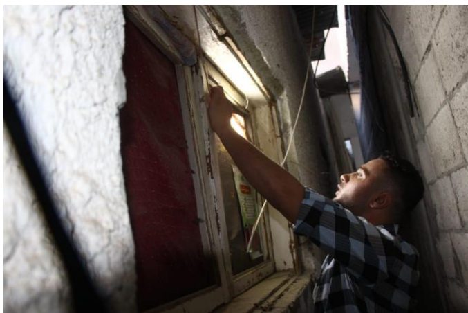
Installing an LED panel
