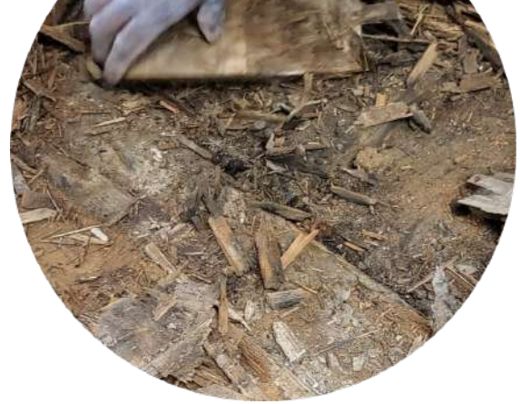
THE COFFEE SHOP FLOOR WAS ROTTEN UNDERNEATH AND HAS NOW BEEN REPLACED
