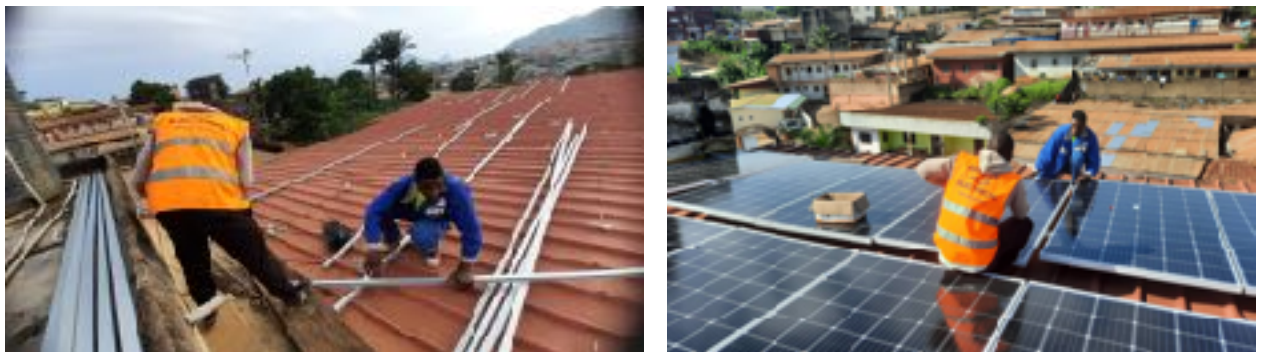
Figure 11 Installing the solar panels with connections to the energy system
