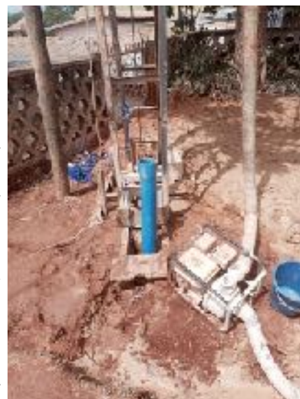
Figure 1 Installing the pipe
