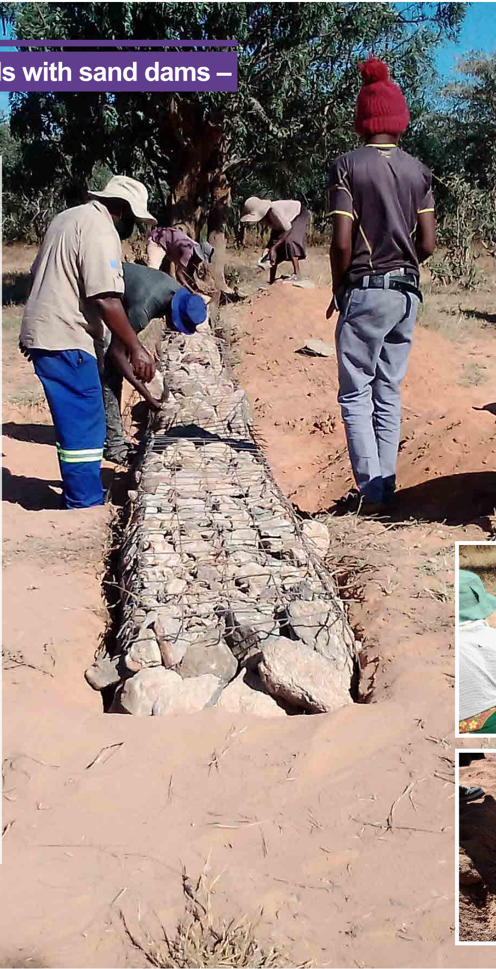
Photos: Stages of stone gabion construction near Nkumbu, Zimbabwe. First there is the digging of the trench and setting out of the wire casing, which is then filled with locally collected stones, before everything is secured with the wrapping of wire.
