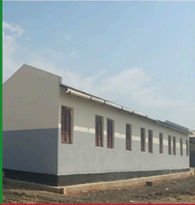
School buildings constructed by WTI, with funding from the Global Partnership for Education
