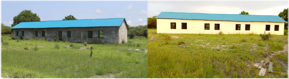
Two classroom block renovations: before and after
