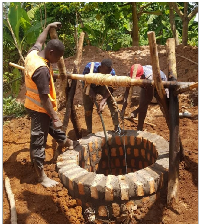
Borehole digging in progress at Buyaga.
