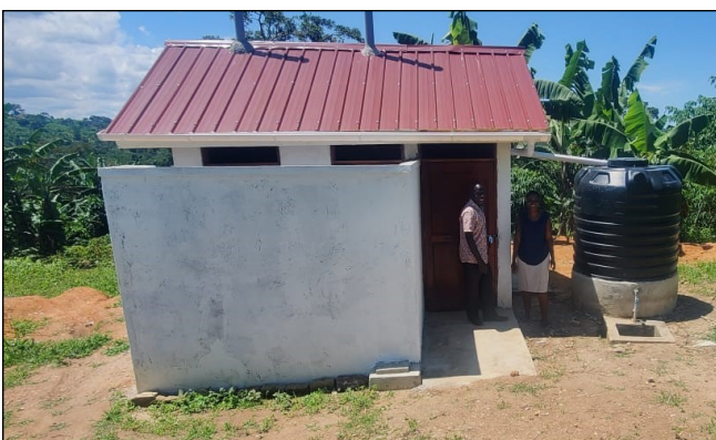
The new accessible toilet block in Nsonga.
