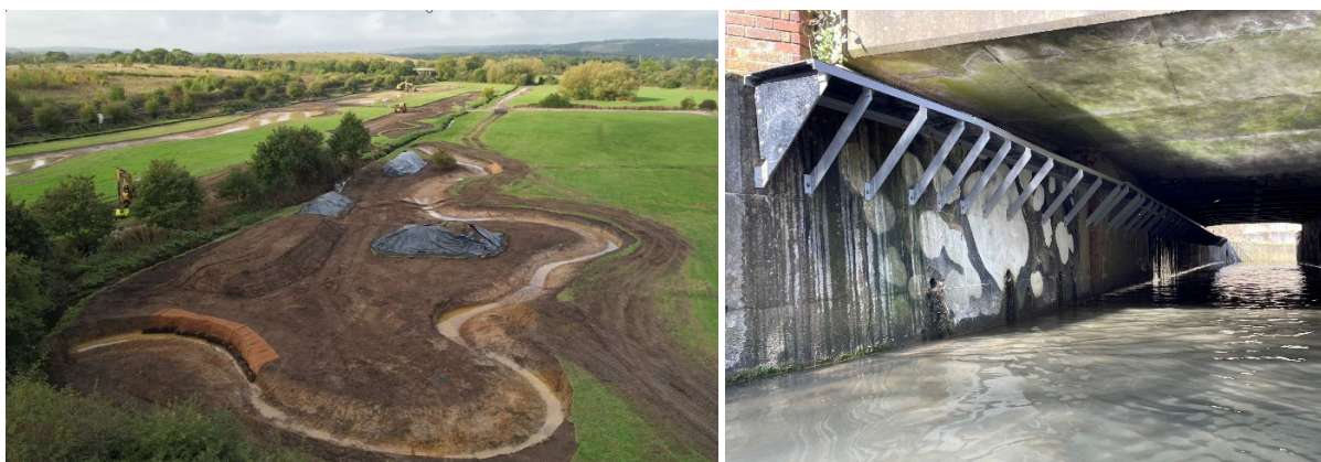
Honeypot Stream restoration (left) as part of South East Water's AMP7 WINEP Adaptive Management Schemes. Work involved building backwaters, habitat enhancements to the existing channel and the creation of three large wetland scrapes. Multi-Species pass (right) underneath the A3 road allowing mammals and other wildlife to access two nature reserves without crossing 10 lanes of traffic.
