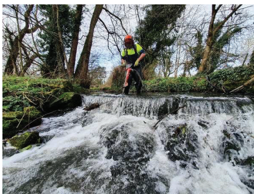
Weir removal on the Darent at Brasted
