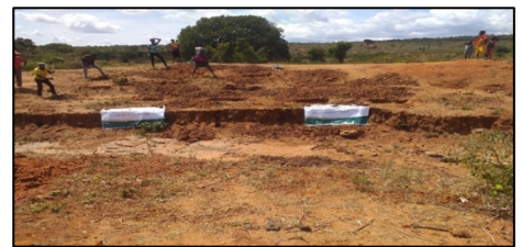
Constructing staggered trenches
