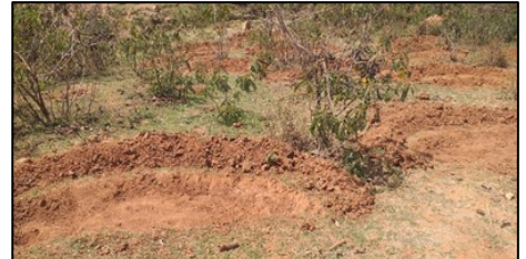
Shaping earth bunds
