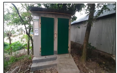
A toilet facility in Narayanganj
