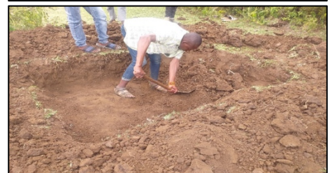
Digging shallow tanks
