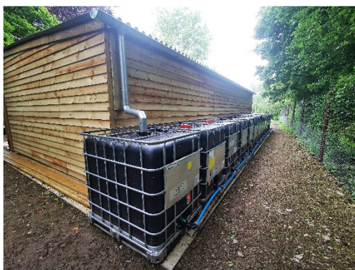
IBC rainwater harvesting at Dartington
