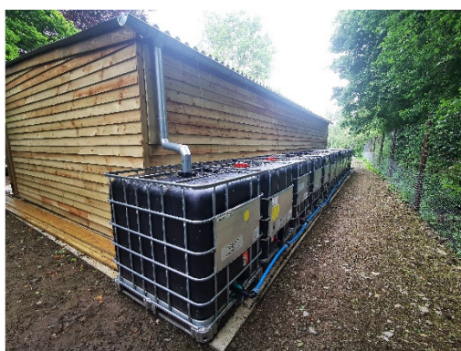
IBC rainwater harvesting at Dartington
