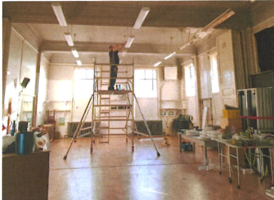
Lighting upgrades in progress
