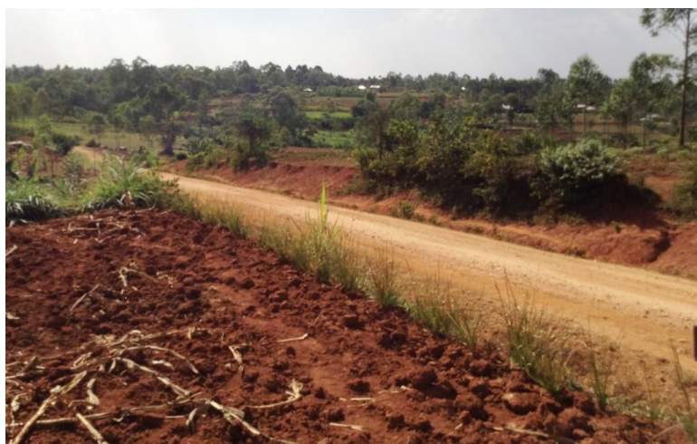
Vetiver Grass planted to protect land by an upgraded road near Butere
