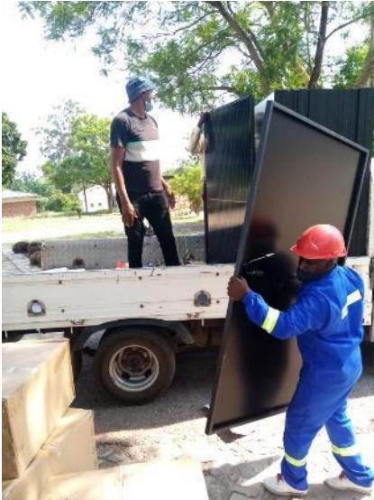
Off loading panels.
