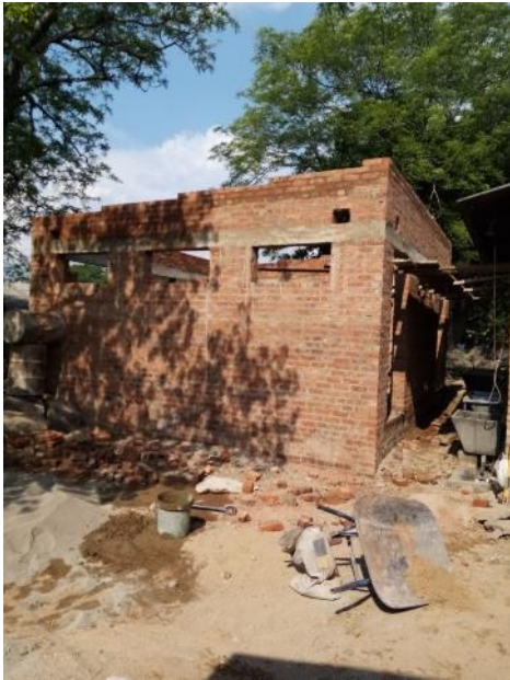
Cooking shelter under construction.
