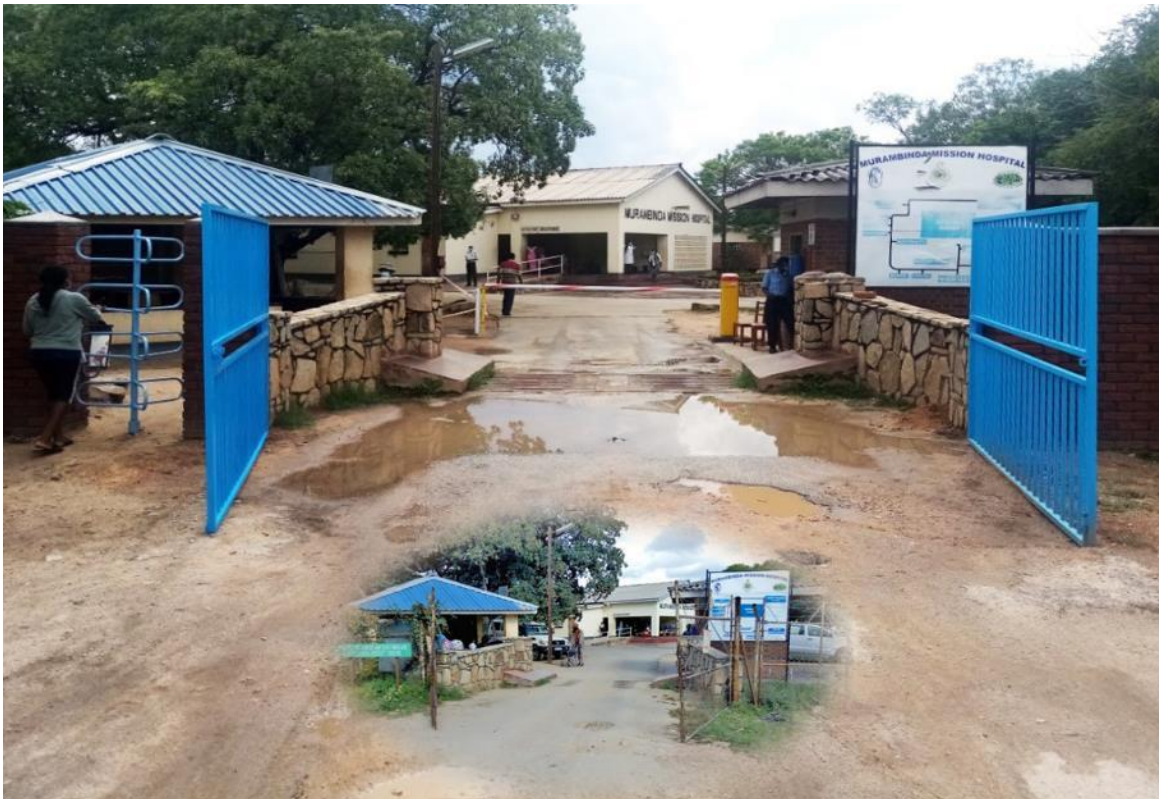
The main hospital entrance renovation completed making for better security.
