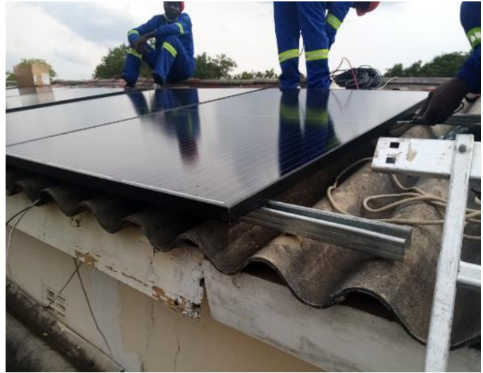
Installation on the pharmacy...
