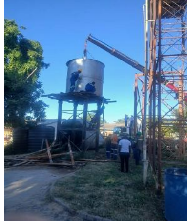
Lifting into place
