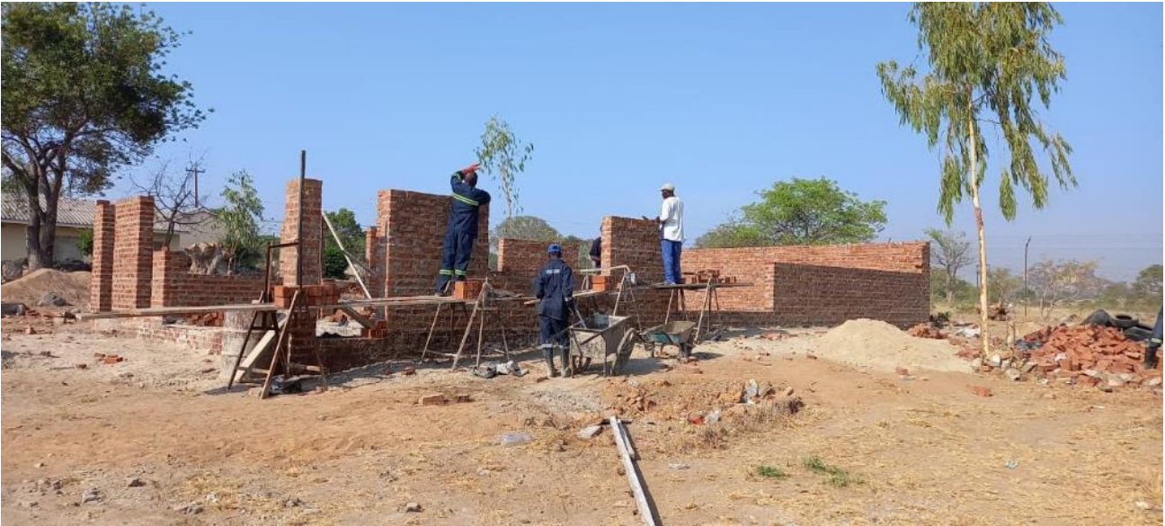
Work in progress November 2022
