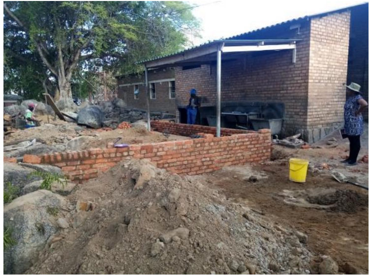
The mothers' shelter under construction.
