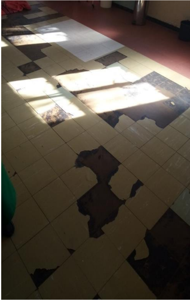
Floor tiles before and after
