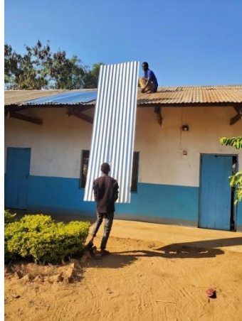
Replacing roof sheets
