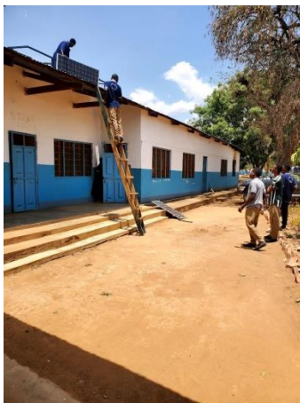
Replacing solar panels
